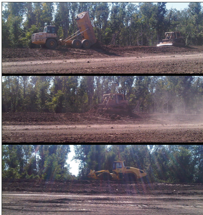
Constructing levee at the lower crevasse. Clay is first dumped (top), then spread to a depth of one foot or less (middle), and finally compacted (bottom). The process is repeated until the levee is at the proper elevation.
