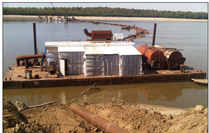
The dredge (background) will pump sand to a booster pump (on barge, center), then to the scour hole at the center crevasse. A flexible pipe section will connect the booster pump to the shore pipeline (foreground).
