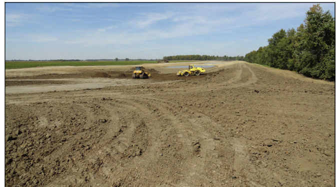
Clay embankment is placed behind the levee at the upper crevasse Thursday to prevent seepage.
