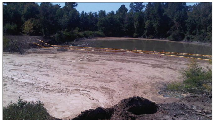
Engineers installed a silt curtain at the center crevasse this week. The silt curtain will prevent silt plumes from entering the existing scour hole (visible in background).
